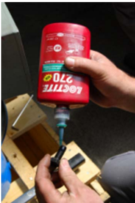
Fig. 35: Apply thread-lock compound to the bolts
